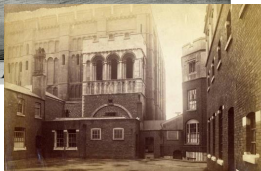
The Castle from the same side in the late 1880s showing prison wings, the turnkey's office and part of the Governor's house.
